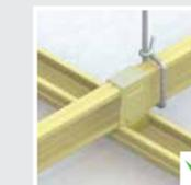
Right: The connection between main bars and cross bars is secure, causing no collapse to ceiling system
